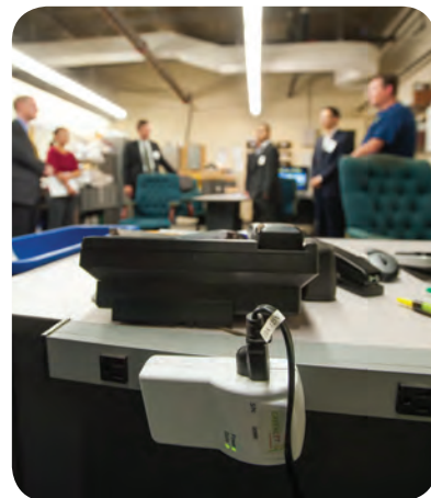
One of 200 Greenlet electrical outlets installed in the School of Engineering's West Hall as part of its microgrid. The outlets help control power consumption by fine tuning the delivery of electricity based on demand. Utility representatives from China toured the facility to learn more about the VCU microgrid.
